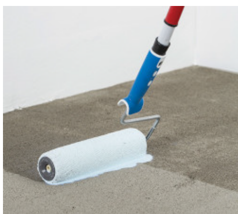
Primer application on the substrate
